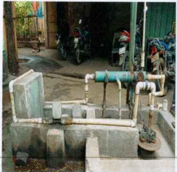
Digital Water Meter in Borewell at gate No. 3
